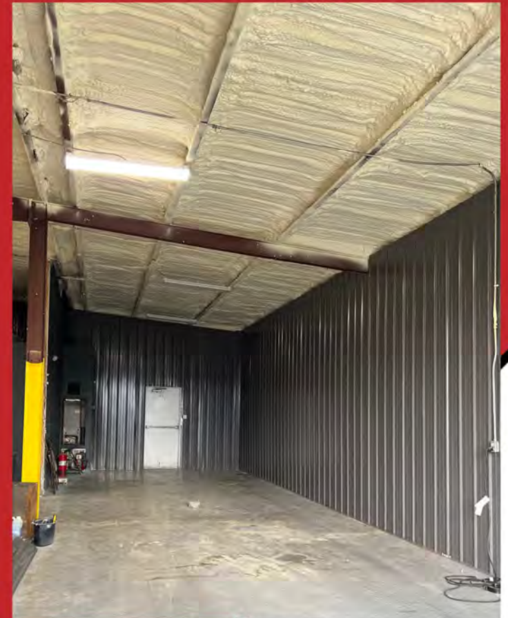
Recent renovations to Meadow Village station
